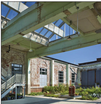
Original building condition. From: Du Toit Architects.
