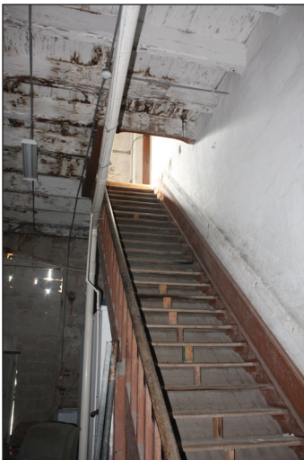
(Top) Freight Elevator, Second Floor. (Bottom) Stair Connecting both floors.
