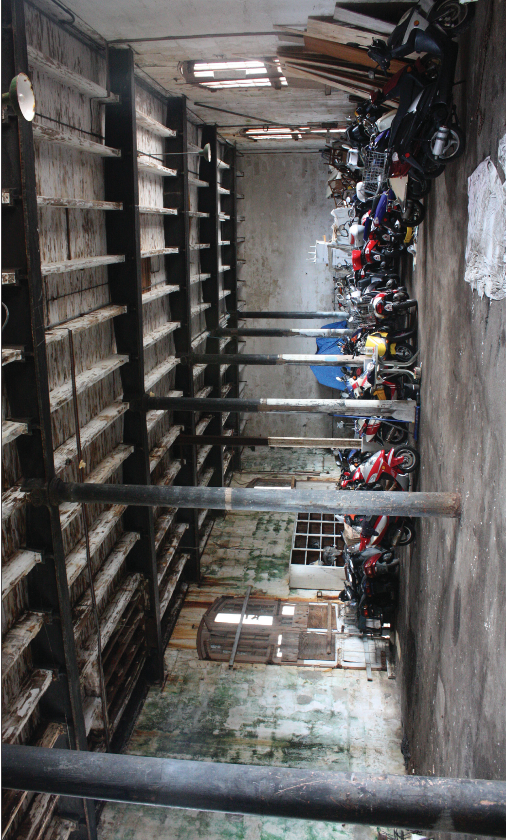
Existing Conditions Storehouse No. 2 today is used for storage of cycles for the nearby rental company. View of the Ground floor.
