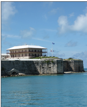
View of Commissioner's House from the water, looking North.
