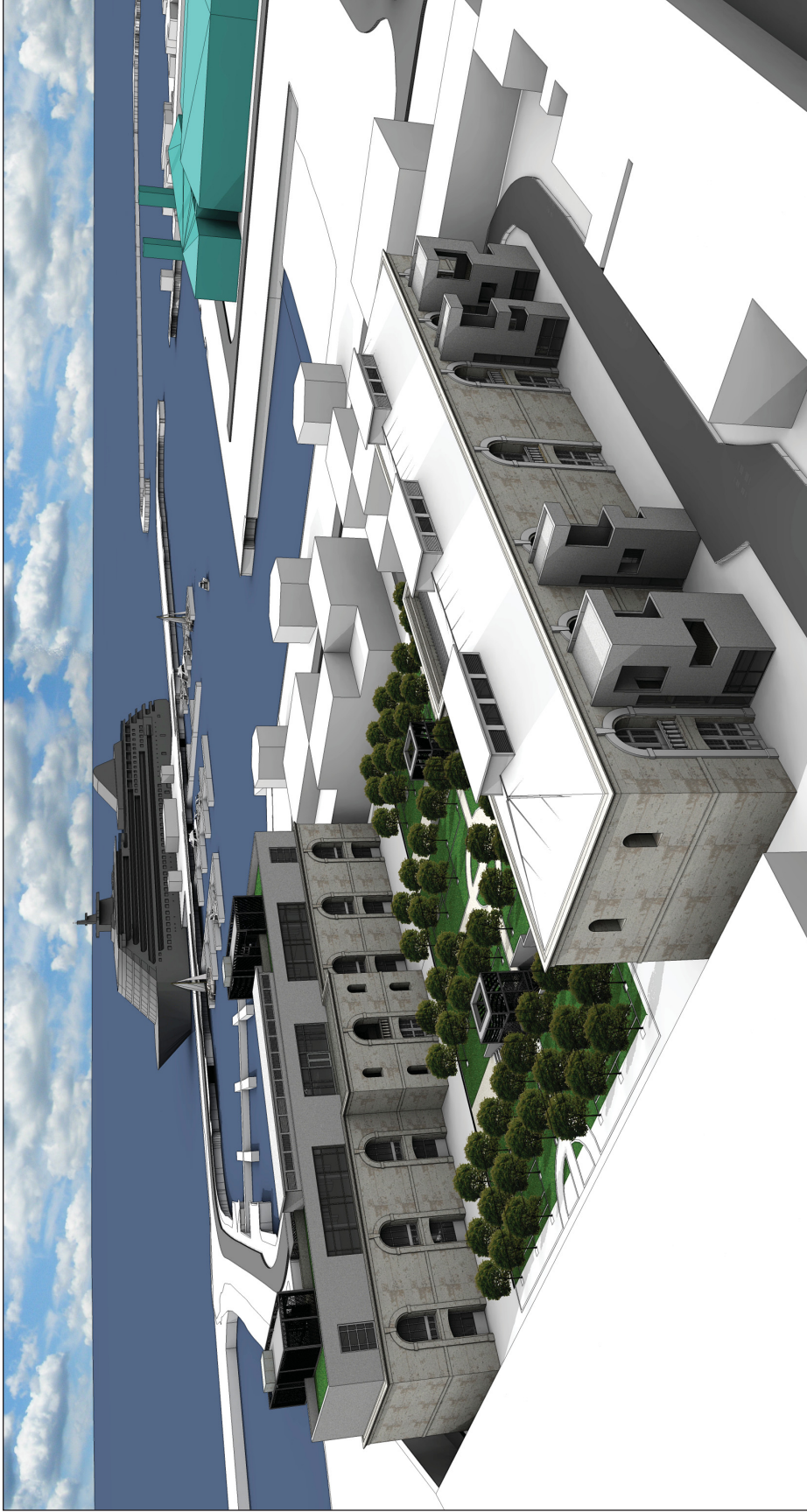
Overall View (Foreground) Artists' Residence. (Background) Art School. Note the addition of the Pilot Project on the back of the Artists' Residence. They will be constructed using reinforced concrete block, and provide supporting services such as: kitchens, bathrooms, and laundry services. Also they are privately accessible balconies for each tenant.
