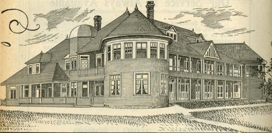
OLD INFIRMARY (Original Building) Nova Scotia Sanatorium
