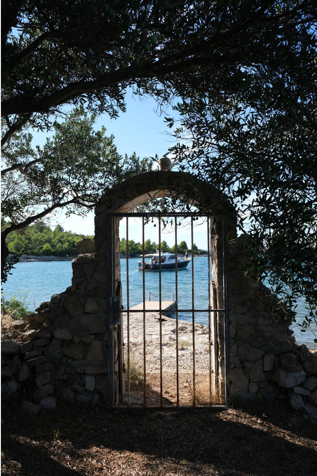
Figure 31. Photograph showing the existing arch and concrete dock on the site.
