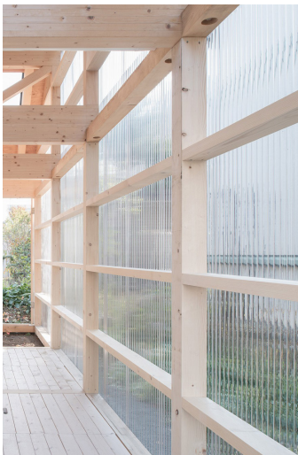
Figure 36. Polycarbonate Wall in a House in Skinkawa by Yoshichika-Takagi Sapporo, Japan (Oseto 2015).
