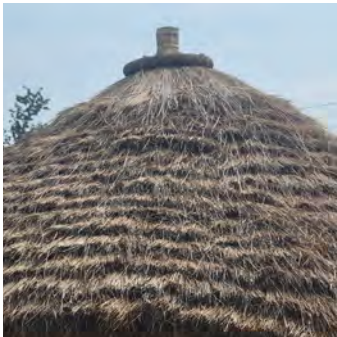
Detail photo of thatch showing layering.
