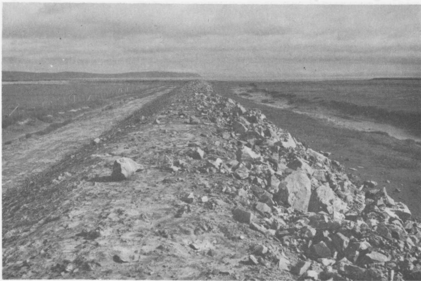
Figure 6 - Grand Pre Marsh, Kings Cumberland County, N.S. - Heavy rock facing on the protecting dyke to avoid erosion by wave action during high tide periods.
