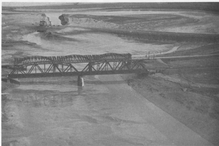
Figure 2 – Tantramar River Dam, Westmorland County, N.B. – The rock-fill dam and water control structure in the background protect approximately 18,000 acres of marshland. In the foreground is the CNR bridge and behind it the old highway bridge.
