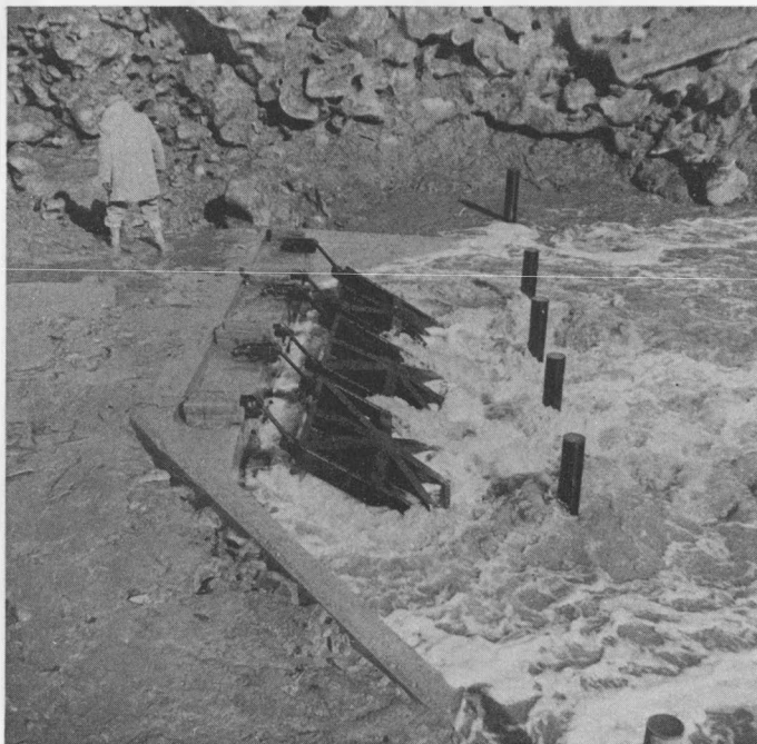
Steel gates discharging a heavy fresh water flow through the sluice at Palmer's Creek, Dorchester Project, after closure in the main fill has been completed. Fill, well above tide height, crosses the sluice to the left. Flow of fresh water ceases when incoming tide reaches the elevation of the fresh water in the reservoir upstream to the structure. March 1956. (Photo N.B. 13//52)
