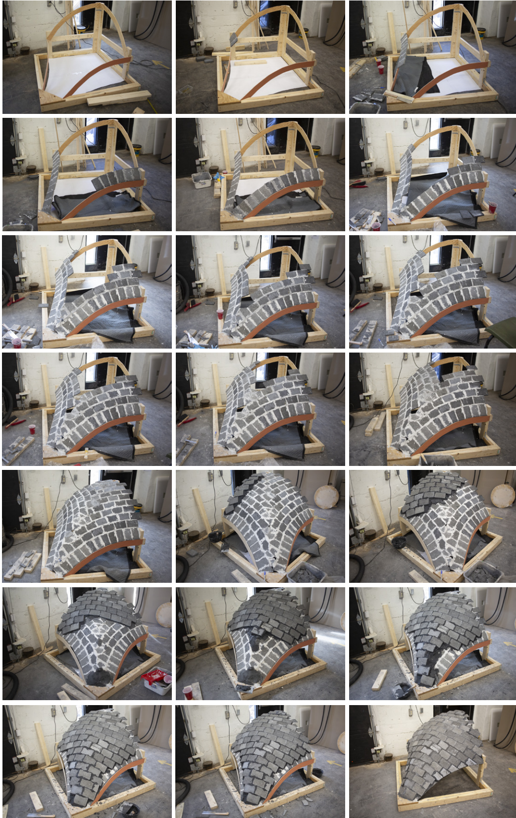
Vault construction process photos
