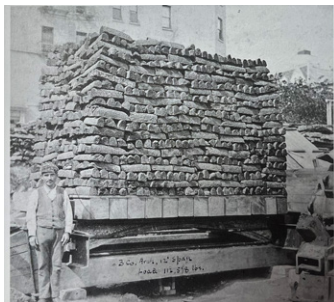
Load test on a tile arch spanning 12 feet that safely carries more than 100,000 pounds (Ochsendorf and Freeman 2010,152)
