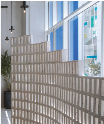
Fig. 54. Bio-bricks assembled into partition screens (Howarth 2022).
