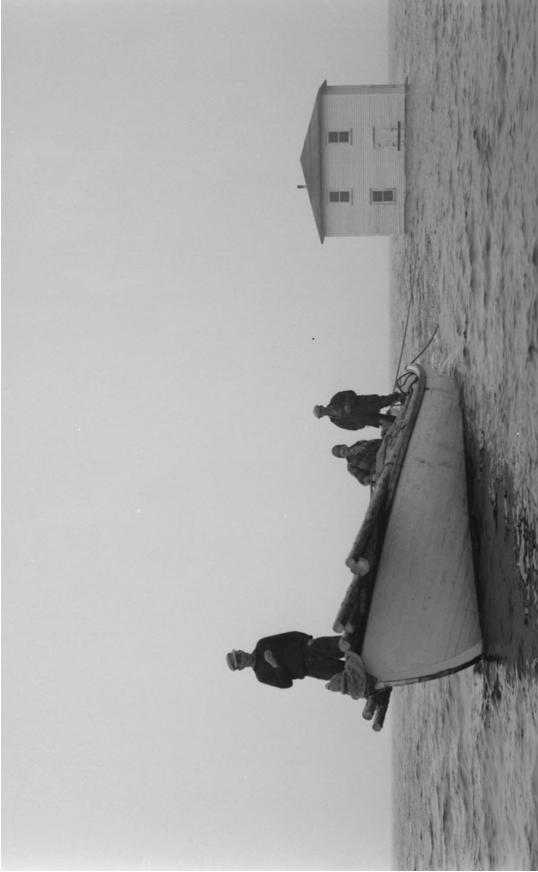
Fig. 5. Photograph of house being floated from an outpost community on empty oil drums to its new location (Town of Dover 1960).
