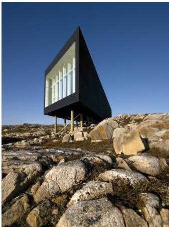
Fig. 15. Long Studio office in Fogo Island (Fogo Island Inn n.d.).
