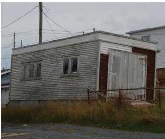
Fig. 32. A shed reconstructed using remnants of old materials.
