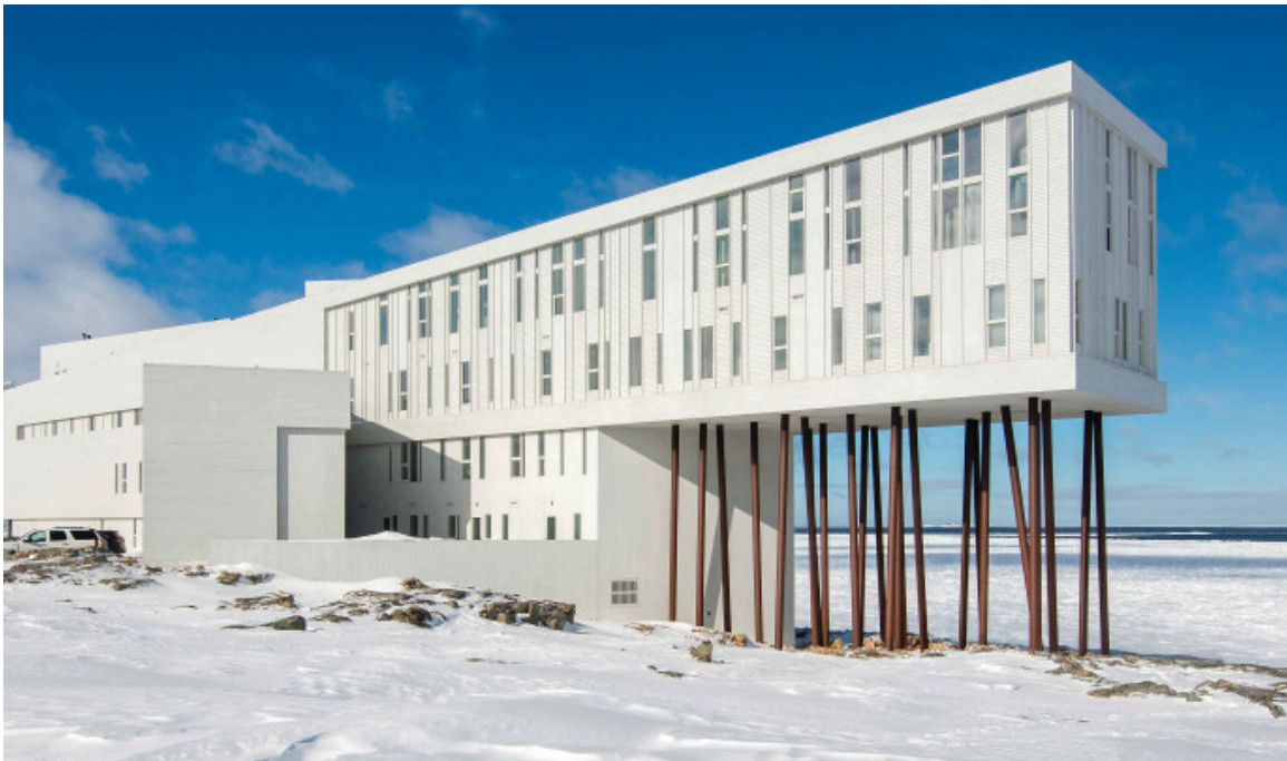
Fig. 12. The X-shaped structure of Fogo Island Inn takes on a modern approach to outpost vernacular, integrating stilts as a distinct feature of fishing stages (Fogo Island Inn n.d.).
