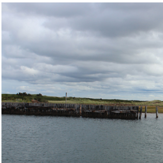
The existing groin infrastructure along the dredged waterway.
