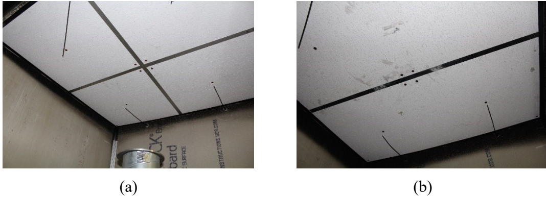
Figure 10 Installed (a) four-tile and (b) two-tile arrangements, viewed from below.
