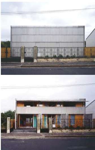
Latapie House. Exterior transformations (Lacaton and Vassal 1993).
