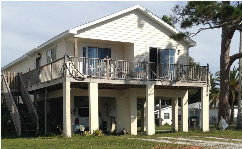
Fig 4 Stilt homes featuring ground level storage and 2 nd floor living areas are becoming more common in coastal and flood prone areas of many southern states (e.g., Florida) (Photograph by author).
