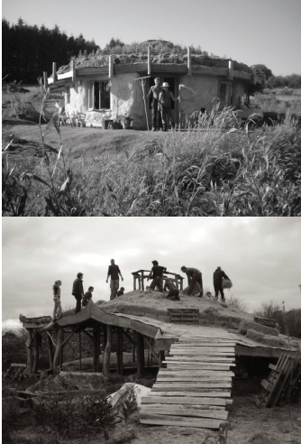
Community natural building at Lammas Ecovillage, Pembrokeshire. Buildings use locally felled trees, straw bale, and cob construction (Lammas n.d.).
