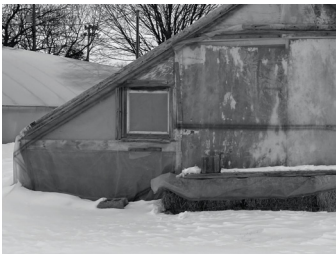
Local precedent for straw bale insulation, on-site, 2020. Local agents place straw-bale around openings of greenhouses during the winter months.
