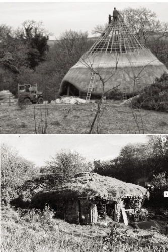
Brithdir Mawr community founded in 1994 (Brithdir Mawr n.d.). Building materials are sourced on the 80 acre property and techniques include thatching with reed and earthen roofs.
