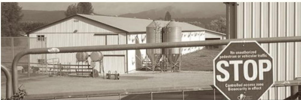
PHOTOGRAPH OF PUBLICLY INACCESSIBLE INDUSTRIAL POULTRY BARN (Cardwell 2020)
