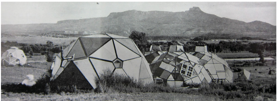
Drop City domes and zomes, 1969 (“In the Spirit of Drop City” n.d.). Salvaged building materials and adaptive techniques lead to creative community efforts, but they also lead to replicable style used by other groups with similar ideology (Macy and Bonnemaïson 2003; Hayden 1976, 399)
