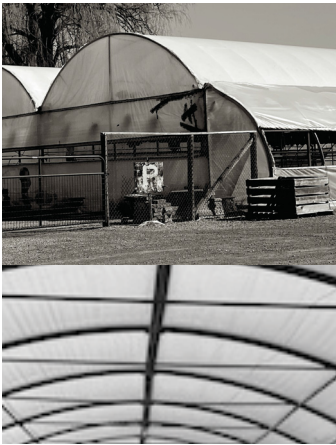
Regional precedent for half arch assembly, Grimsby Ontario, 2020. Commercial greenhouse quonset arches are often assembled using a half arch and connected with a steel ridge beam. This makes for easy adaptation and proliferation of studio types.
