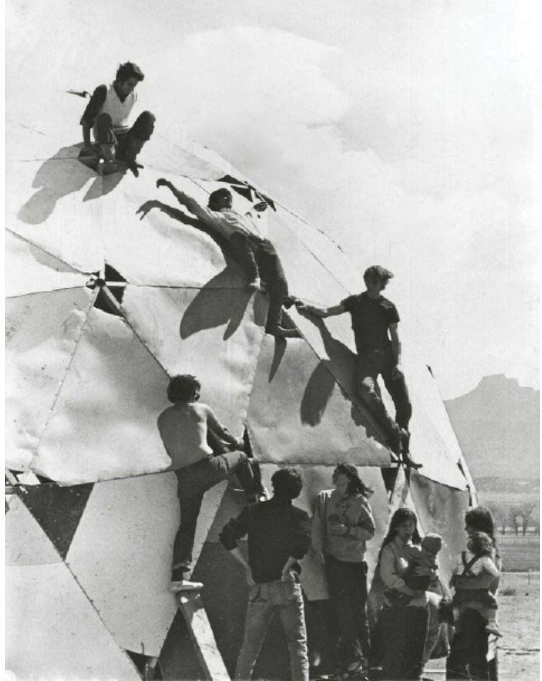
Photograph of dome building process (Sadler 2006). Domes were picked up by the “counterculture” back to the land communes in the 1970s. They came to symbolize nature, critique on global interdependency and consumerism, and closing the loop in architecture in that “nature and culture were inextricably intertwined” (Macy and Bonnemaïson 2003, 325)
