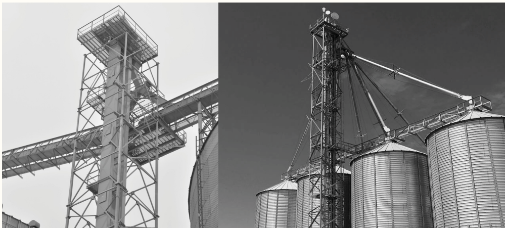
PHOTOGRAPHS OF INDUSTRIAL GRAIN LEG AND SUPPORT TOWER (Whitcomb Brothers Grain Systems Inc. n.d.).
