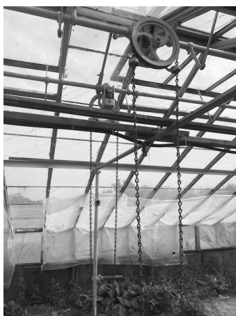
On-site precedent of chain-operated ventilating gear, 2021. In this greenhouse, the hand-wheel was removed to leave the center space clear for carting in and removing soil.
