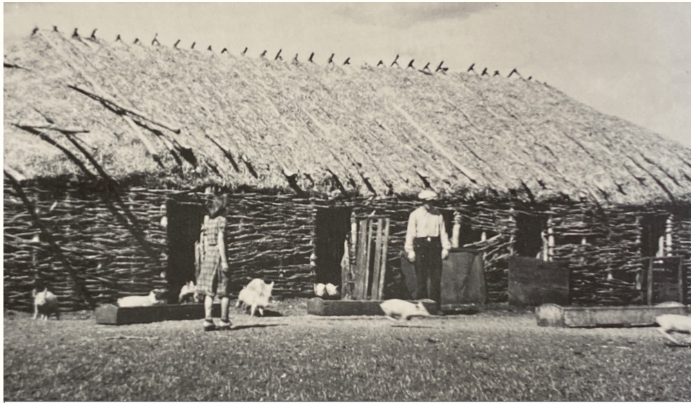
CONSTRUCTION USING REGIONALLY AVAILABLE MATERIALS: EARTH PACKED FLOOR; HEAVY THATCH AS INSULATOR FOR WINTER AND SUMMER; WALLS OF COB, WILLOWS, WATTLE AND DAUB (Arthur and Witney 1972, 10).
