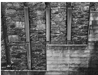
The American method of lock building used a combination of wood slats and local stones. This image was taken at the site of Lock 3.
