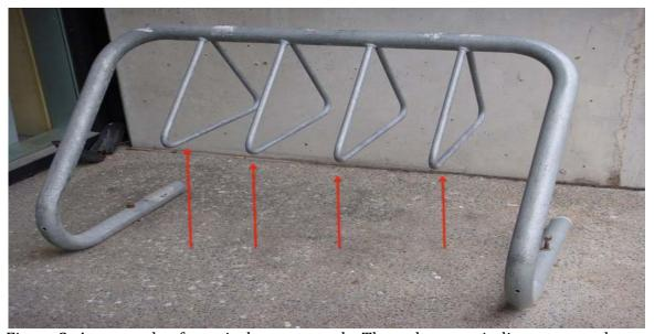
Figure 2: An example of a typical campus rack. The red arrows indicate spots where the researchers assumed that one bicycle could be stored. Thus, for all campus racks the capacity was determined by counting each hoop extension.
