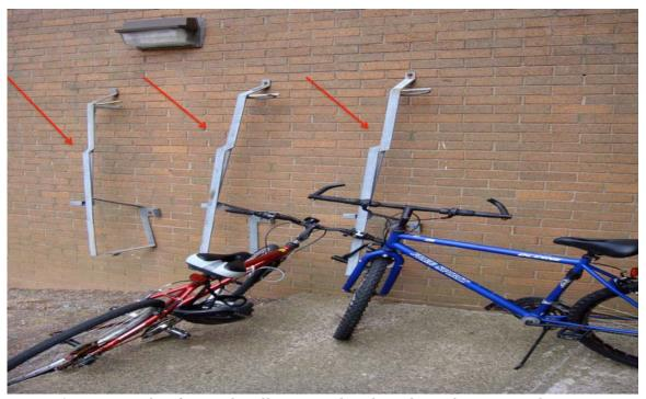
Figure 5: An example of typical wall-mounted racks. The red arrows indicate spots where the researchers assumed that one bike could be stored. Thus, for all wall-mounted racks the capacity was determined by assuming that each wall-mounted rack could support one bike.
