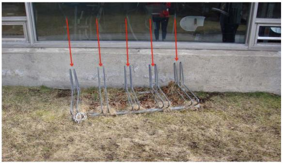
Figure 4: An example of a typical comb rack. The red arrows indicate spots where the researchers assumed that one bicycle could be stored. Thus, for all comb racks the capacity was determined by assuming that each parallel section could support one bike.
