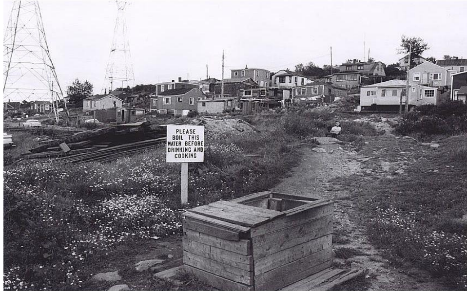
FIGURE 13: AFRIVILLE WELL. THE COMMUNITY DID NOT RECIEVE MUNICIPAL SERVICES. BROOKS, CA. 1965.
