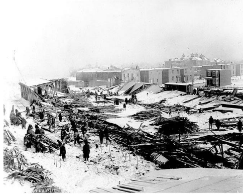
FIGURE 11: COLLAPSED BUILDINGS (NS CAR WORKS) ON CLIFTON ST., HALIFAX. GAUVIN & GENTZEL, 1918.
