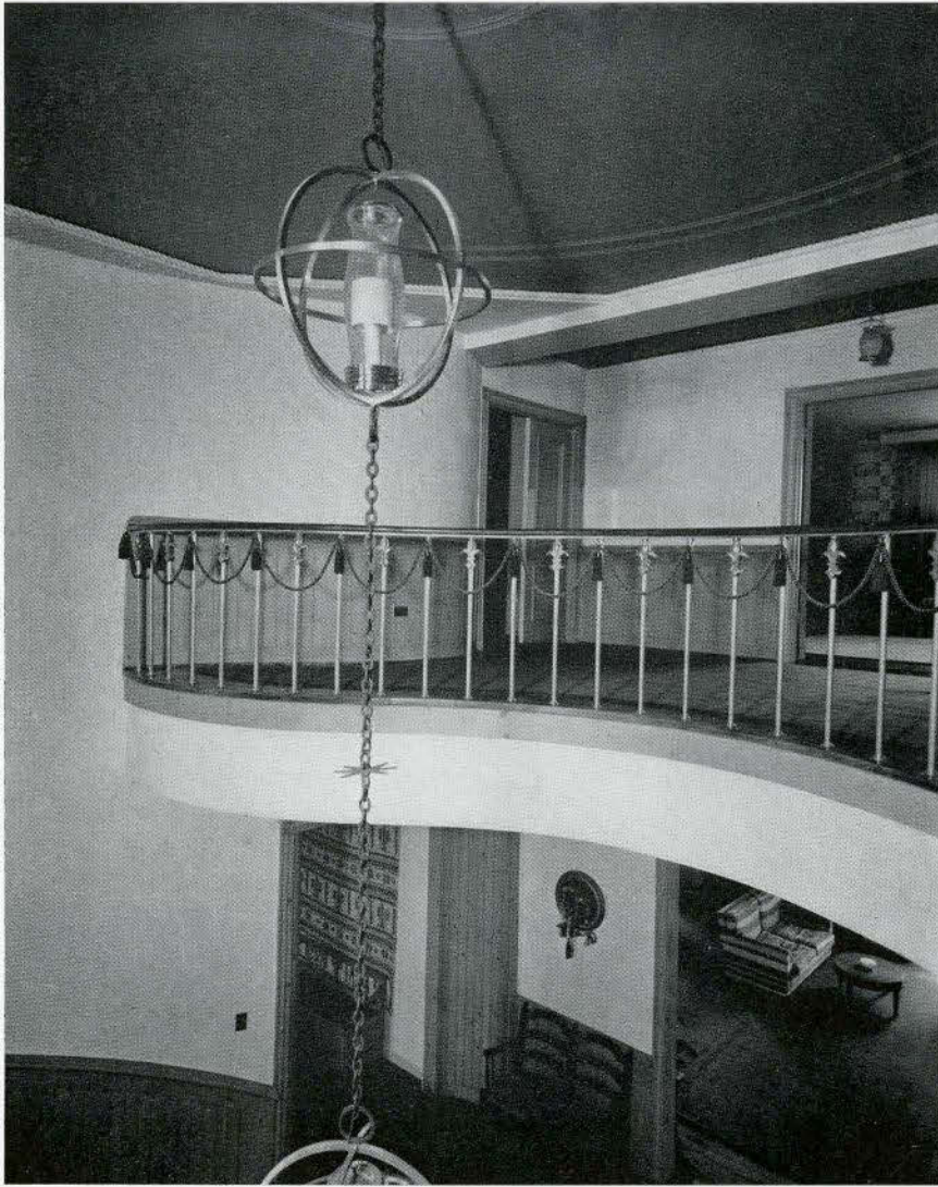
MAIN STAIR. ALUMINUM BALUSTERS AND LIGHT FIXTURES
