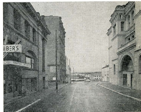
The students, in their study of Old Victoria endorse the recommendations of a 1967 study by Acres Western Limited on renewal for the area – the influence of the already-developed Bastion Square (before and after photos right) should be expanded. They further suggest that a series of "paths" or pleasant walkways should link "places" or activity spaces.
