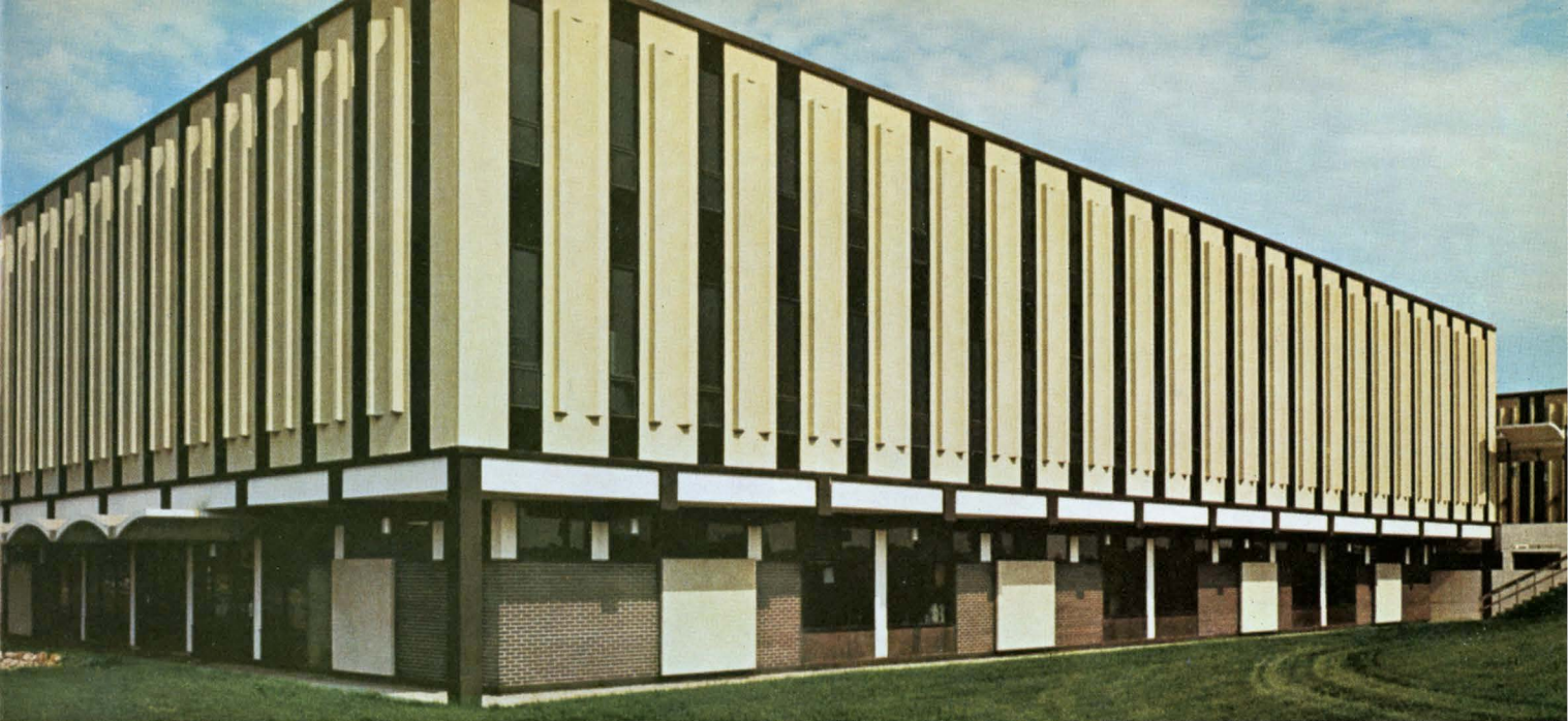
3. Slick and slender precast concrete panels accentuate the vertical lines of the Collège St-Joseph, Université de Moncton, N.B., reflecting its dynamic spirit.
