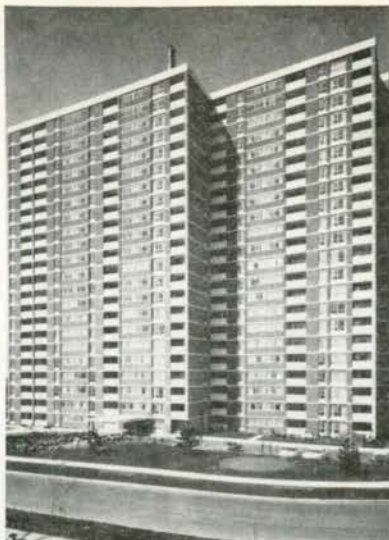
"Top of the Valley" Apartment Complex, Toronto, Ont. Owners: The Rubin Corporation & Mr. Jos. Godfrey. Architects: Henry Fliess. Consulting Structural Engineers: Reicher Bradstock & Associates Ltd. General Contractor: The Top of the Valley Limited. Masonry Contractor: Zachary De Vuono. Concrete Masonry Blocks: Richvale Block Supply Co. Ltd. Ready-Mixed Concrete: S. McCord & Co. Ltd.
