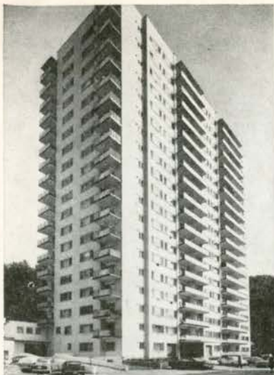
The Forest Hill Apartments, Montreal Owners & Builders: Raoul Blouin Ltée. Architects: Charles Grenier. Consulting Structural Engineers: G. Horvath & Associates. Masonry Contractor: U. Tomassini & Frères Ltée. Ready-Mixed Concrete: Francon Limited.
