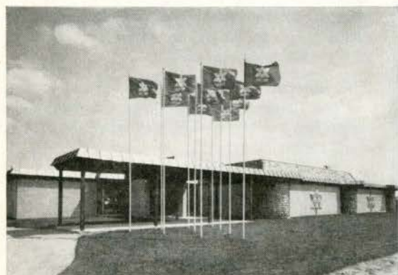
Columbus Centre, Kitchener, Ont. Owners: Corporation of the Knights of Columbus. Architects: Horton & Ball. Consulting Structural Engineers: McCargar & Hachborn Ltd. General Contractor: Brandon General Contractors Ltd. Masonry Contractor: Seibel Masonry Ltd. Concrete Masonry Units: Forwell Ltd. Ready-Mixed Concrete: Albert Raith Cement Contractor Ltd.
