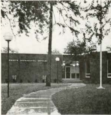
Essex Municipal Building, set among trees on the main street.
