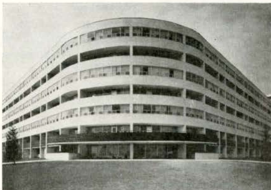
Markham-Eglinton Square, Toronto, Ont. Architects: Martin L. Mendelow. Consulting Structural Engineers: Farkas, Barron, Jablonsky. General Contractor: F.T. Developments Ltd. Masonry Contractor: M. Rodaro Co. Ltd. Concrete Masonry Units: Meteor Building Supplies Ltd. Ready-Mixed Concrete: Mel-Mix Concrete & Asphalt.
