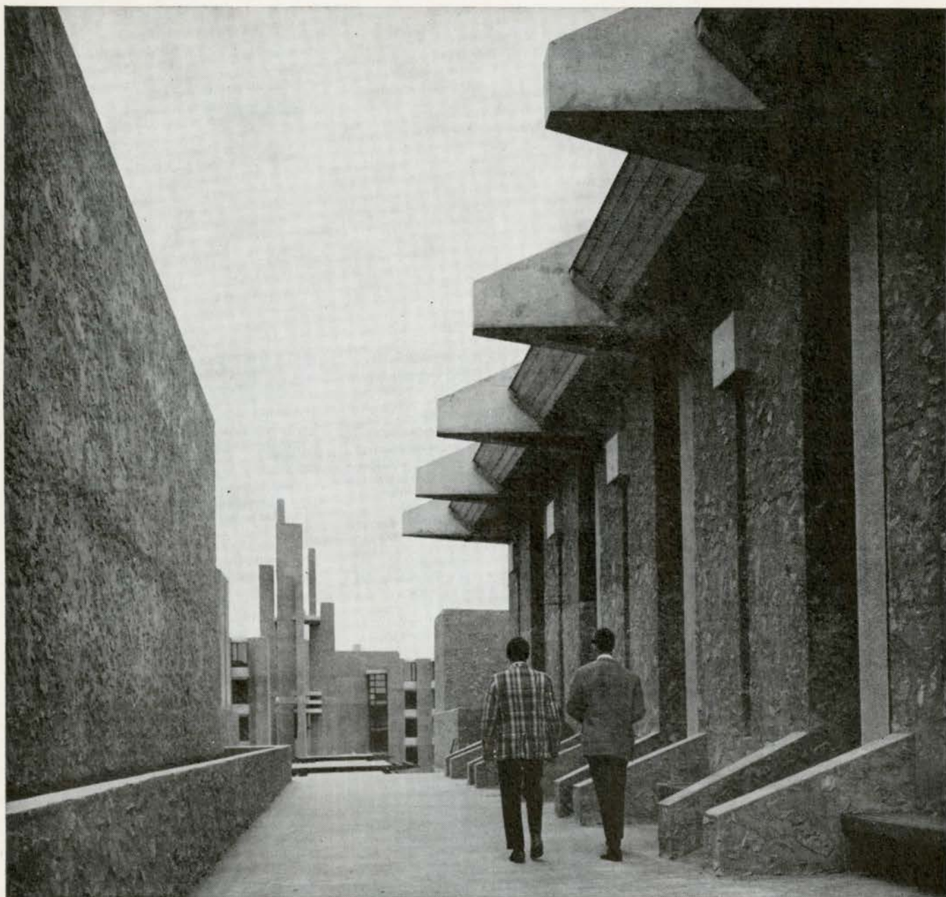
Champlain College, Trent University, Peterborough, Ontario Architect: Thompson, Berwick, Pratt and Partners, Toronto Structural Engineer: M. S. Yolles Associates, Ltd., Toronto
