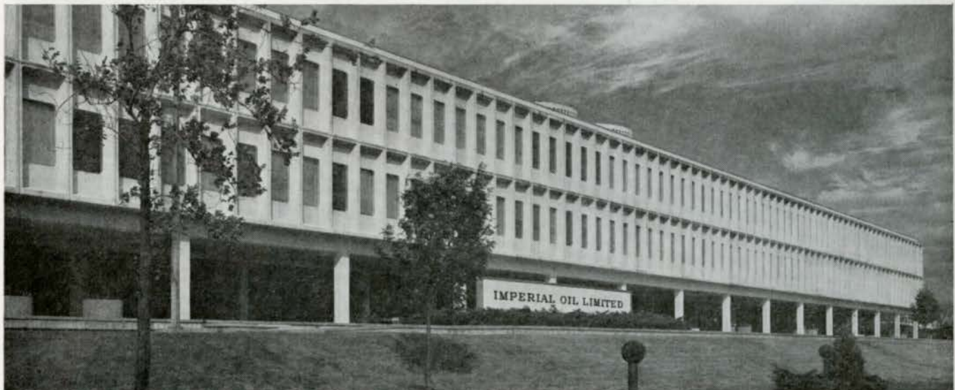
Imperial Oil, Ltd., Toronto. Architect: John B. Parkin Associates, Toronto. General Contractor: Eastern Construction Co., Toronto.
