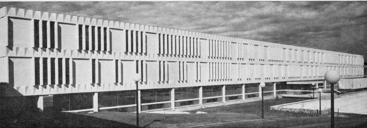
Arts and Humanities Building
