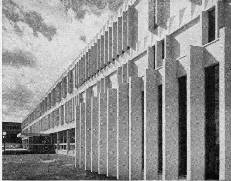
Arts and Humanities Building.
