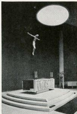
Unusual altar treatment in bush-hammered concrete.
