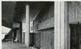
Classic, massive, sturdy concrete columns and wall.
