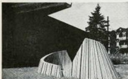
Roof-drainage trough and well, in cast-in-place concrete.
