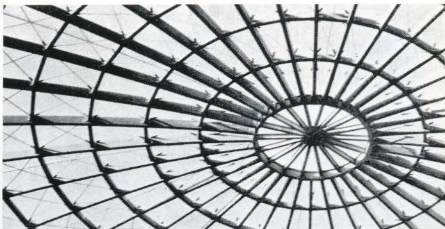
Field House, Montana State College, Bozeman, Mont. Illustration from Shell Architecture.
