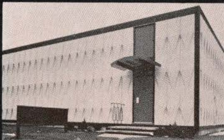
Bell Telephone Dial Building Architect: H.D.L. Morgan
