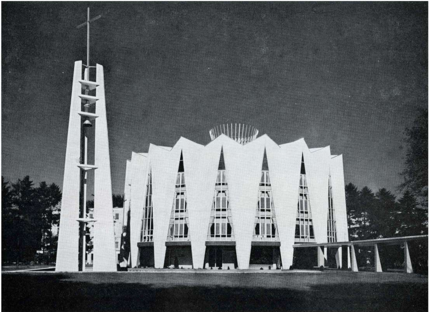
This circular chapel, notable for its precast concrete columns and roof, is the focal point of the Pines, a complex of buildings erected to mark the centenary of the Ursuline Sisters in Chatham, Ontario. Architect: Joseph W. Storey. Consulting Structural Engineers: Todgham and Case in association with Edgar A. Cross & Associates. Contractor: Eastern Construction Co. Ltd., Windsor, Ont. Supplier of ready-mix concrete: Watson Concrete Products, Chatham, Ont.
