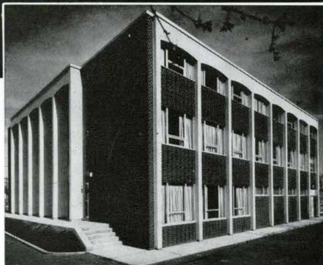
MAGISTRATES COURT BUILDING, Willowdale, Ont. ARCHITECT: Sproatt and Rolph GEN. CONTR.: Stowe and Gould Ltd. PRECAST PANELS BY: Pre-Con Murray Ltd.
