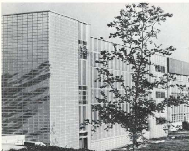
... in commercial buildings
