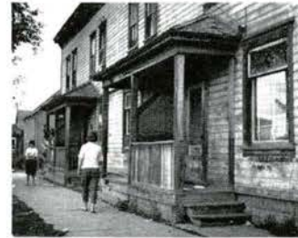
Condition of buildings
