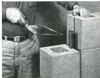
Two engineered products that meet a need. Dur-o-wal reinforcement, shown above, and Rapid Control Joint, below. This ready-made control structure flexes with the wall. Recommended by construction engineers especially for concrete block.
