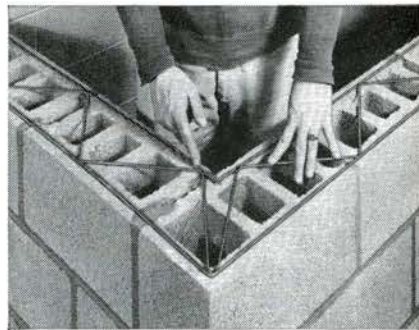
Two engineered products that meet a need. Dur-o-wal reinforcement, shown above, and Rapid Control Joint, below. This ready-made control structure flexes with the wall. Recommended by construction engineers especially for concrete block.
