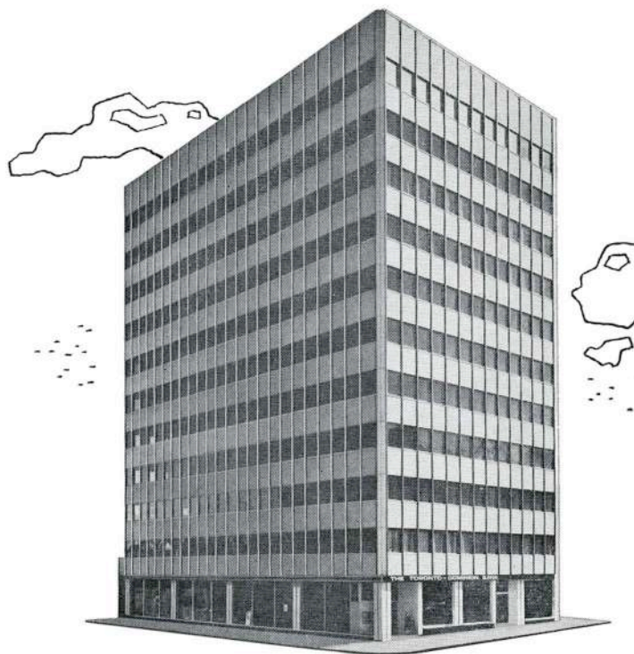
• PRECAST CONCRETE CURTAIN WALL WITH MO-SAI® SPANDREL PANELS AND GRANUX® MULLIONS, 1420 SHERBROOKE WEST, MONTREAL ARCHITECTS: PETER DICKINSON & ASSOCIATES
