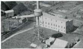
1 Located centrally in the Ajax Development this "furnace" is capable of supplying plentiful heat—or steam—to buildings within 2-mile radius with total coverage of over 16 square miles
