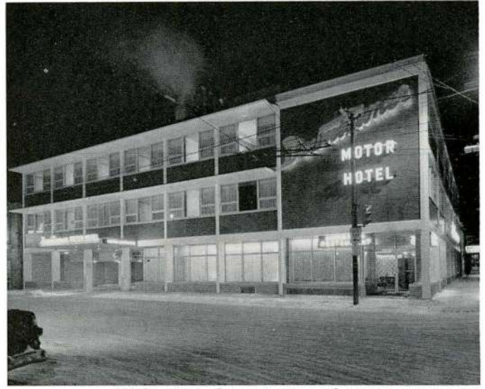
Night view showing car and restaurant entries
