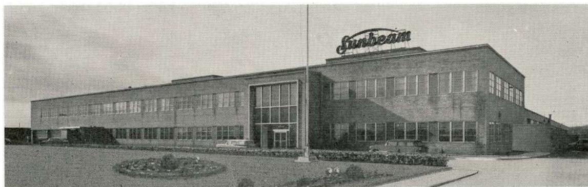
Sunbeam Corp. (Canada) Ltd. Mechanical Contractor, Beaver Engineering Co.
