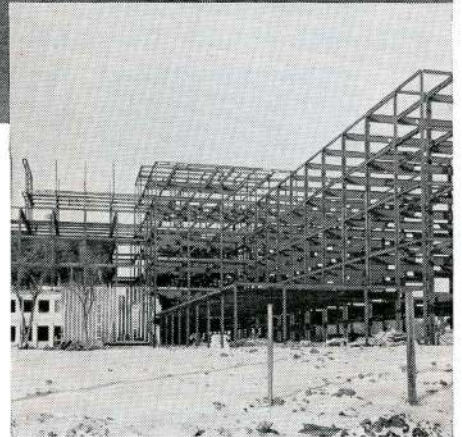
1800 tons of steelwork, fabricated and erected by Dominion Bridge, Winnipeg. Most of this was of "rigid frame" design.
