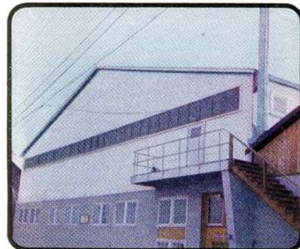
Fish Packing Plant: B.C. Packers Ltd., Vancouver, B.C. Building Designer: Owner Aluminum Fabricator: Nesco Aluminum Ltd.
