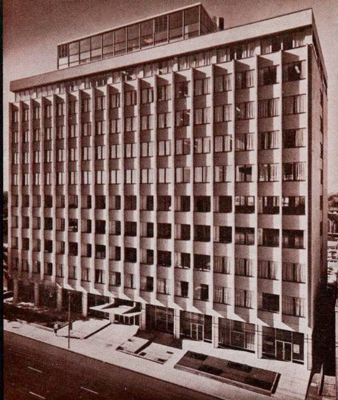
• MO-SAI CURTAIN WALL, 150 EGLINTON EAST, TORONTO ARCHITECTS: PETER DICKINSON & ASSOCIATES
