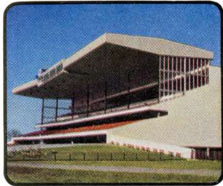
Race Track Grandstand & Clubhouse: Ontario Jockey Club Ltd., Malton, Ont. Architect: Earle C. Morgan Aluminum Fabricator & Erector: Robertson-Irwin Ltd.
