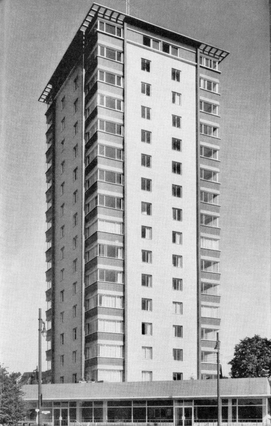
BERKELEY TOWERS, Vancouver. POZZOLITH was a definite help in achieving the excellent finish of this building. ENGINEER: Robertson, Kolbeins, Teevan & Gallaher. ARCHITECT: Polson & Siddall. CONTRACTOR: John Laing & Son (Canada) Ltd. CONCRETE: Deeks-McBride Ltd. TESTING: G. S. Eldridge & Company, Ltd.
