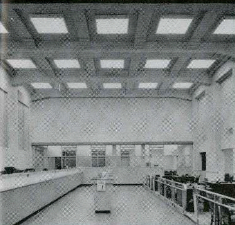
Trust Co.: 4 ft. Square Surface-Mounted Luminaires
