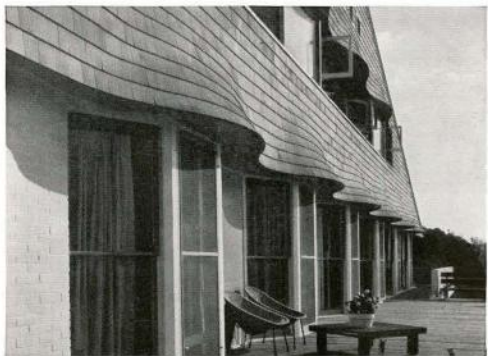
Architects answer a tough design problem—give interesting weather protection to beach home where all rooms have windows facing seaward. Answer: a fresh design motif suggestive of rolling surf—undulating “eyebrows” of weathered silver-gray wood shingles.
