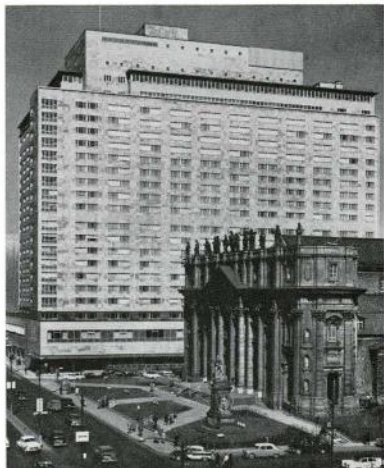
Architects, C.N.R. Staff First under George Drummond, Chief Architect Later under his successor, Harold C. Greensides Architect in charge of the project, John W. Wood
