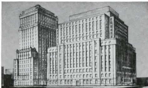
MONTREAL, 620 Belmont Street Building Architects: BAROTT, MARSHALL, MERRETT & BAROTT Engineer: McDOUGALL & FRIEDMAN Air Conditioning Contractor: LONG-ABOUD LTD. Heating Contractor: TWEDDLE LTD.
