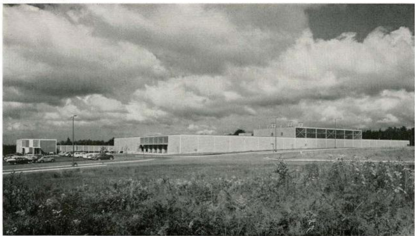
General view of plant
