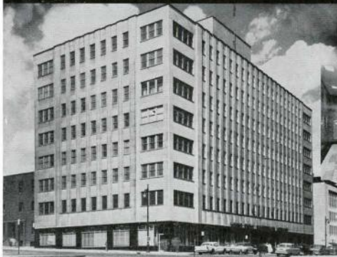
MONTREAL, Canadian Overseas Telecommunication Corp. Building Architect: A. LESLIE PERRY, Montreal Consulting Engineers, Mechanical: JAMES P. KEITH & ASSOCIATES General Contractor: RICHARD and B. A. RYAN, Montreal Heating Contractor: JOHN COLFORD CONTRACTING LTD., Montreal Air Conditioning Contractor: CANADIAN COMSTOCK CO. LTD., Montreal
