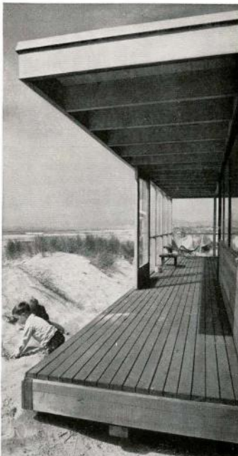
How to have your beach house on the sand, but not in it—set the house on wood piles several feet above the dunes, provide generous walkways of separated wood strips to filter out tracked-in sand. Note generous frame overhang, vital for sun protection.
