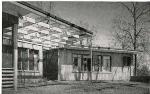
Simple, patterned wood overhang provides dramatic focal point at little cost—because it's of wood. Changing shadow pattern adds interest to patio, filters sun's intensity without cutting light in adjacent dining area.
