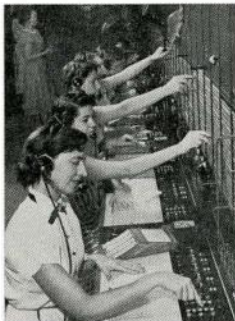
Proper temperature control helps avoid mistakes, as in this direct-dial long distance switchboard room.
