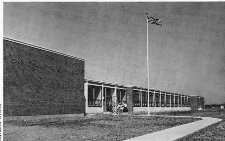
Architects, Burgess and McLean
