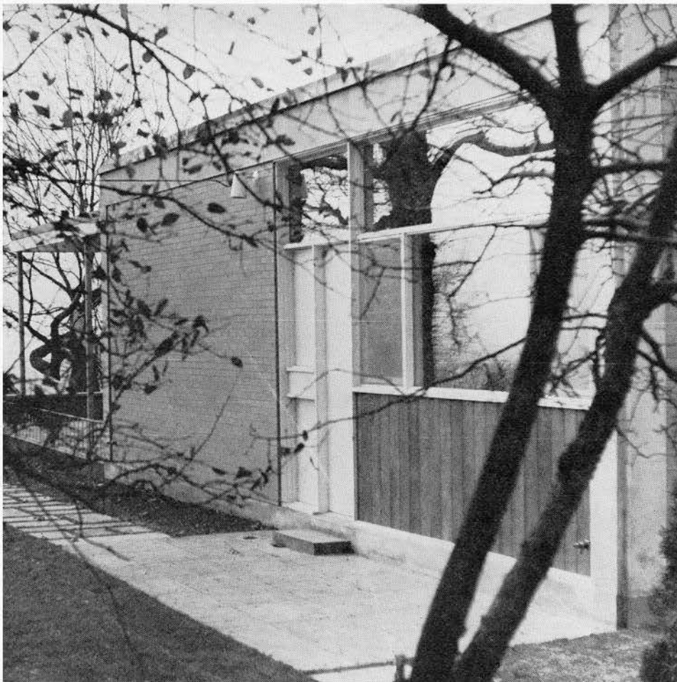
Detail of corner of south elevation
