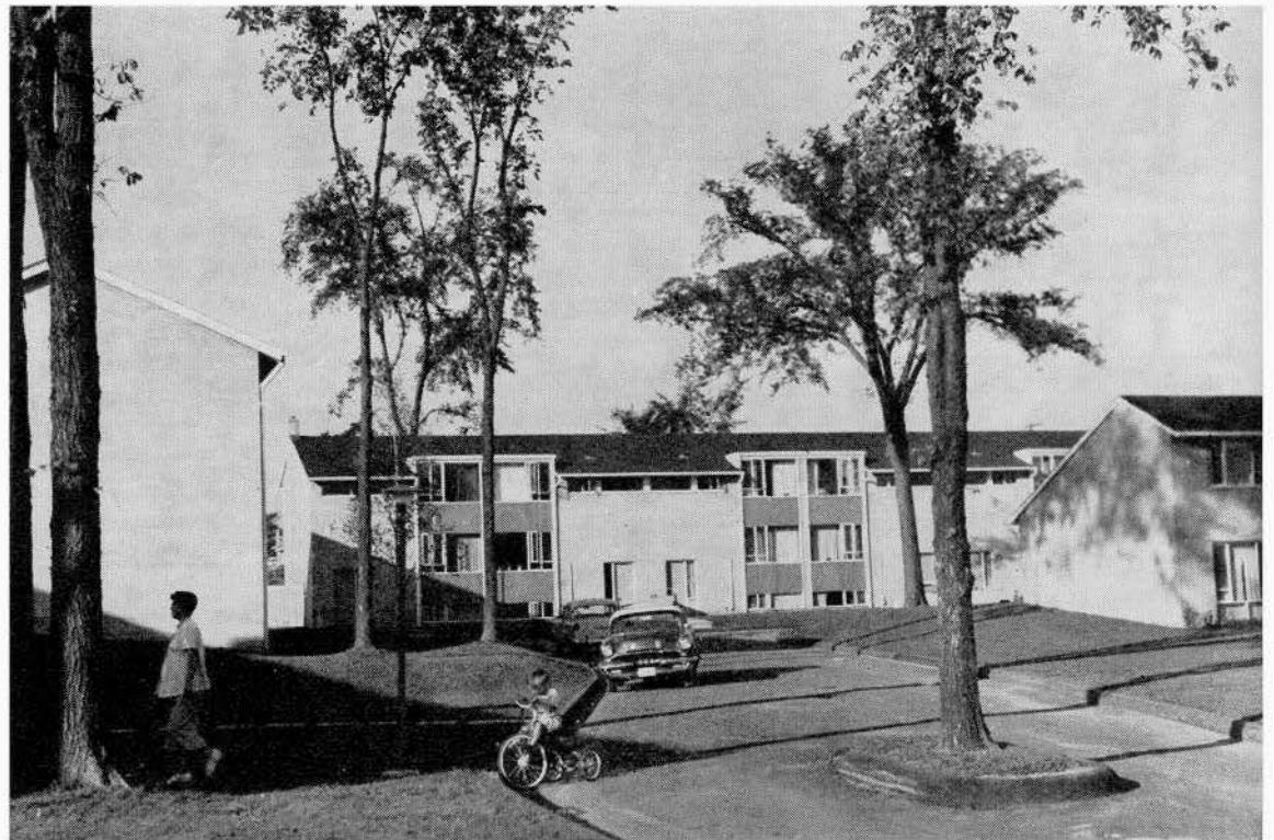
View showing the front elevations of the two-storey unit
