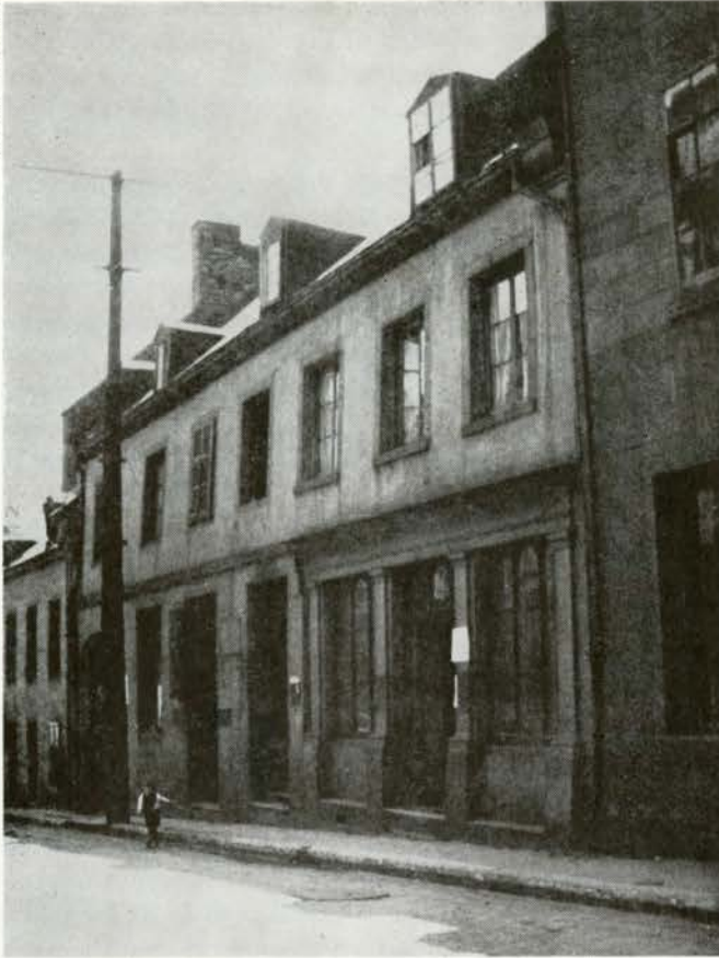
A house on St. Vincent Street in Montreal, now destroyed. It is of the type of the early nineteenth century, although it could be older. The lower floor appears to have been altered to accommodate quite a pleasant shop in the manner of the Royal Engineers. The lower and possibly later alteration, which consisted in making a window into a door is more un-gainly. The wall is rubble masonry thickly plastered. The margins of the windows and corbels for the parapets are cut stone.
