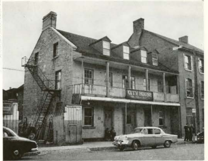
City House, Murray Street
