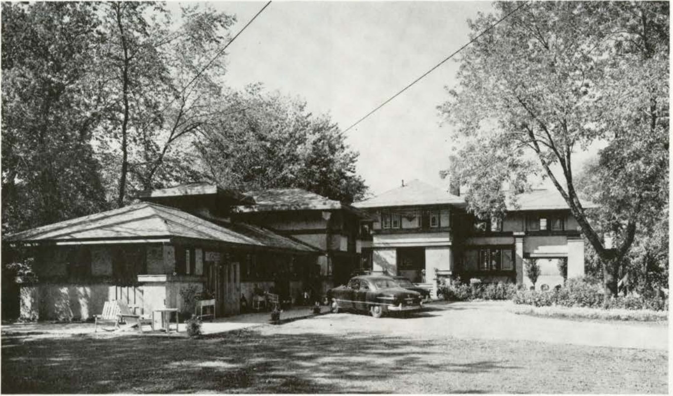
Gorman House, Woodroffe Architect, Francis Sullivan
