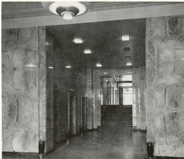
Ground floor interior
