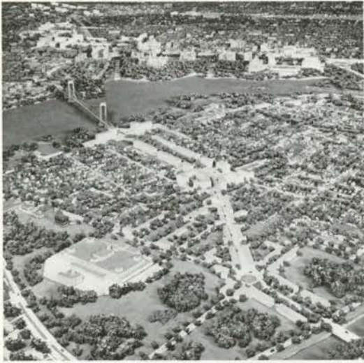
The eastern section of Hull with the Capital across the Ottawa River to the south. The new Government Printing Bureau is seen left centre. The boulevard running from the bottom of the picture to the bridge will be constructed on what is now the CPR right of way.
