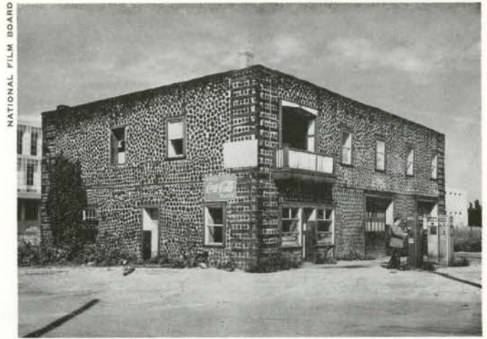
Short log construction, Hull
