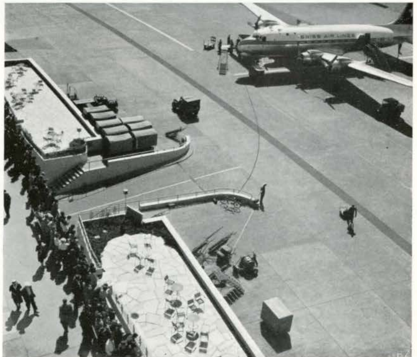
The splayed parapet of the entrance to the baggage floor (basement) of the Passenger Wing. During winter the part of the tarmac immediately before the entrance is heated to keep it free from snow.
