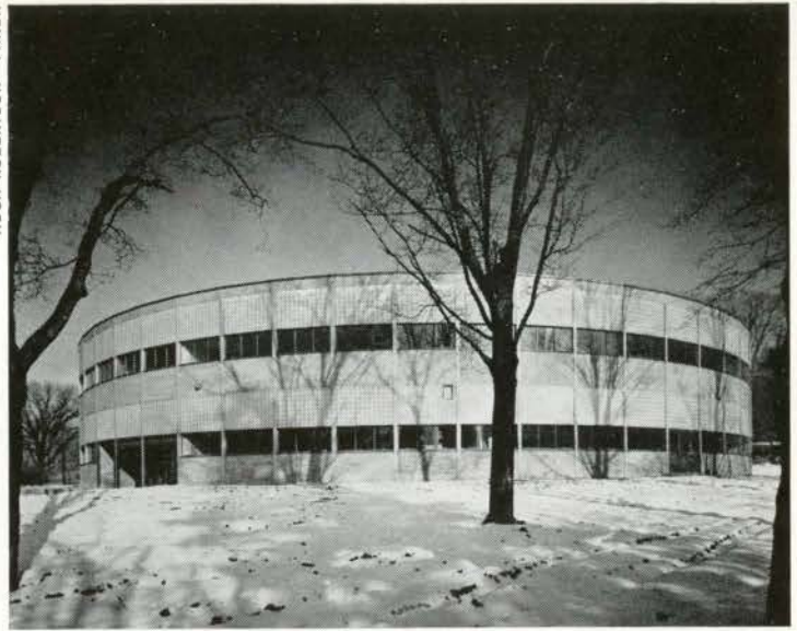
View from the south-west on Ninth Street. The main structure is two storey, sixty-sided, with brown-grey steel columns exposed, steel plate fascia, and copper coping and drip. Solid in-fill panels are of local light red brick. Steel sills and sash are painted charcoal grey.
