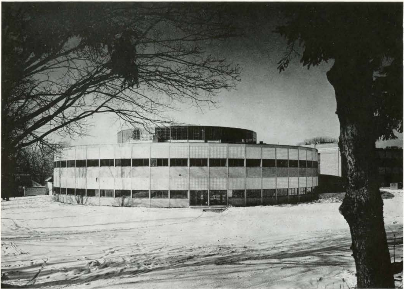
View from the south-east hill showing gymnasium clerestorey and the separation from 1925 Vocational Wing.
