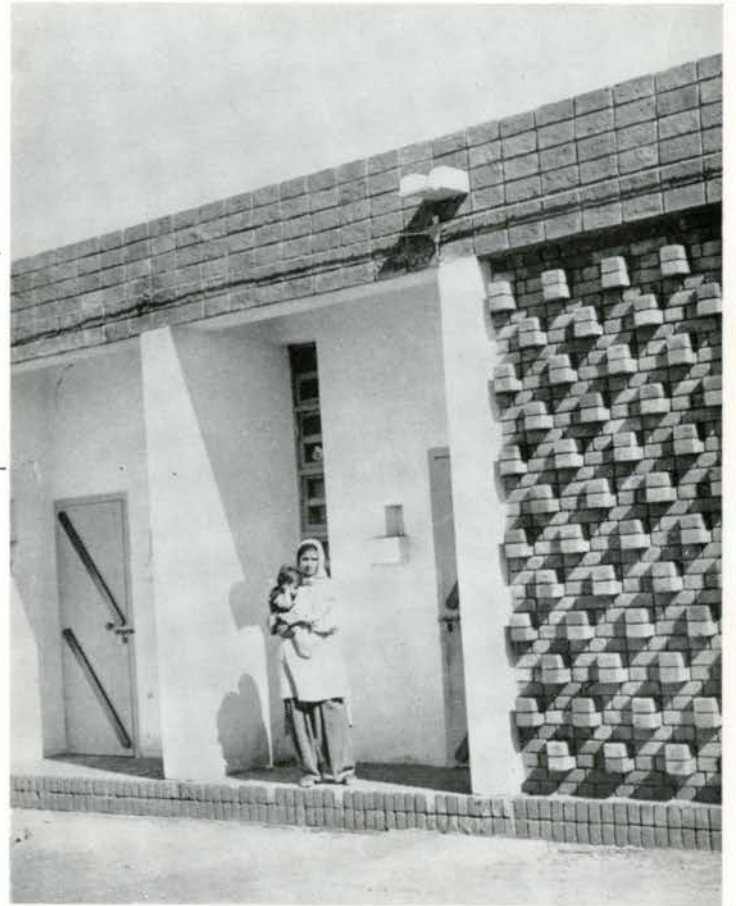
Entrance. Note patterned wall always in half shade and projecting water spout from flat roof.
