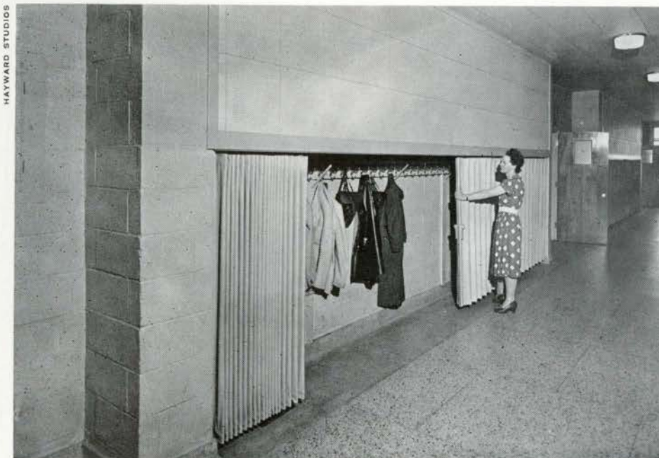
Corridor wardrobe unit
