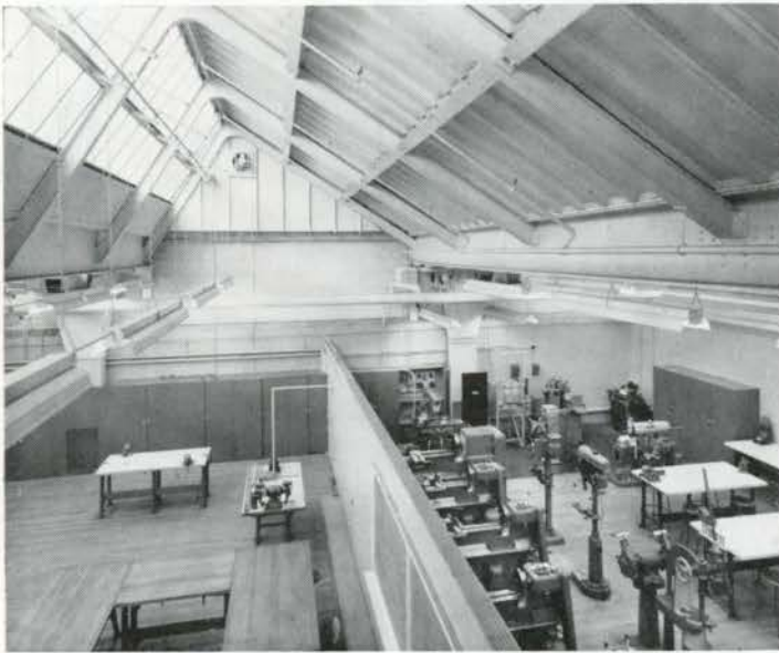
View looking down into east half of shops area from gallery over administration and draughting centre core area.
