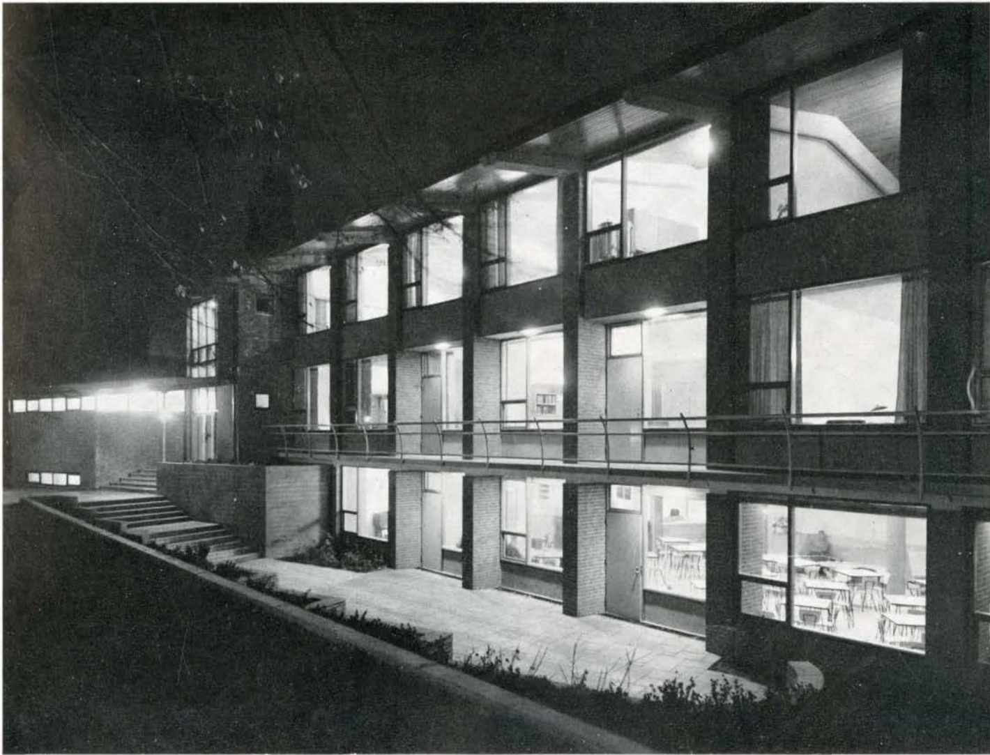
The main building at night. A continuous grille-covered drain at the wall takes care of run-off in the lower court. Perimeter insulation was omitted here to keep the drain open in winter. The continuous balcony simplifies window cleaning and shades coffee shop windows.
