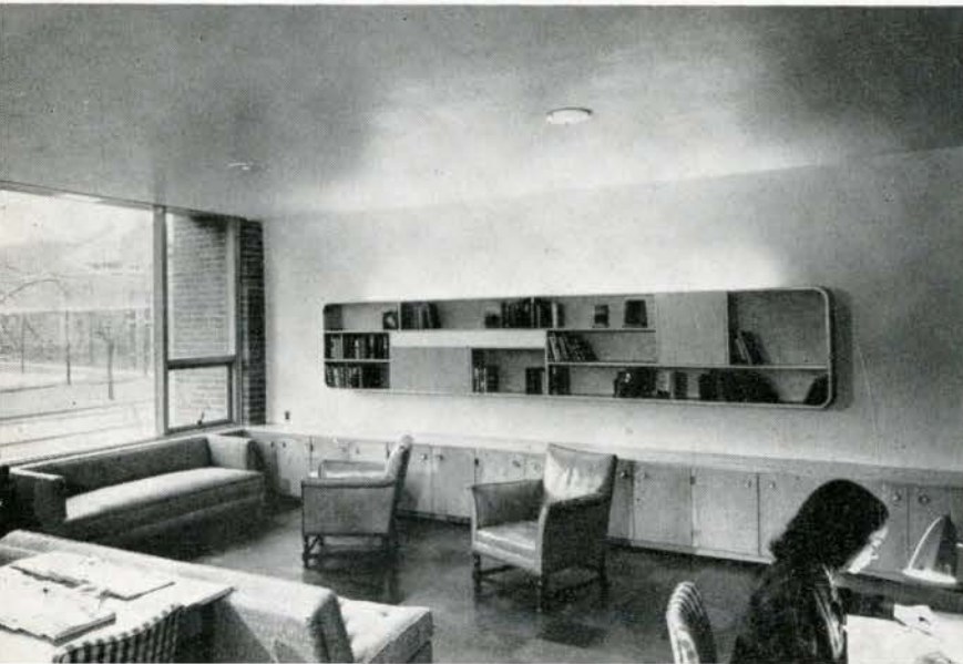
The reading room has a furred ceiling to accommodate kitchenette piping above. In most rooms piping is concealed in masonry. The floor is cork tile.
