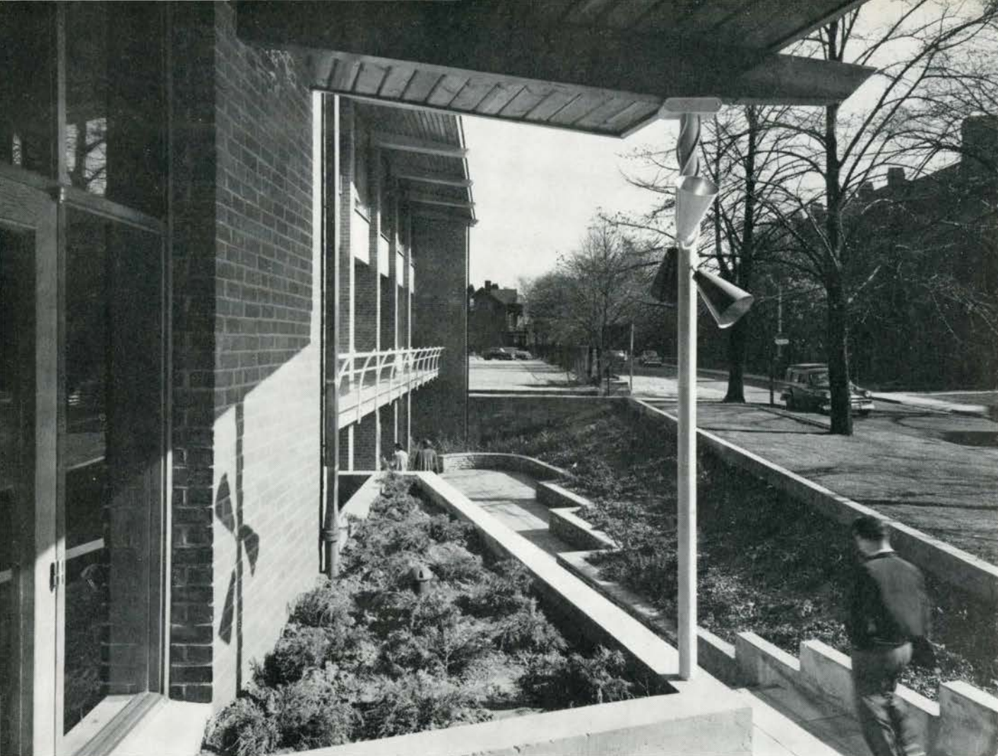
The sunken garden from the main entrance. A dry stone wall and sloping bank planted in evergreen groundcovers accommodate the change in grade from street.
