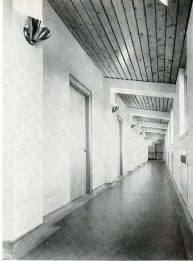
Third floor corridor shows typical construction: exposed concrete columns and beams, exposed haydite block, linoleum floor with terrazzo base and border.
