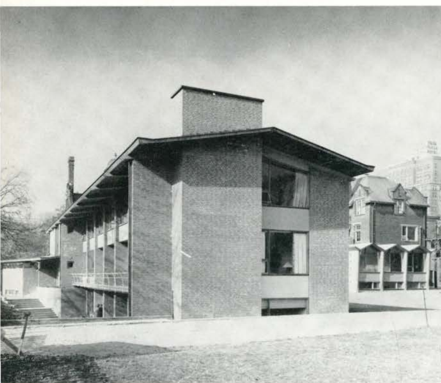
The main building from the east shows the typical structure, load bearing masonry walls, precast concrete spandrels, concrete beams and plank roof.
