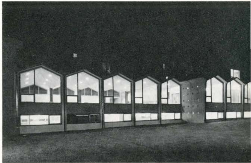
The cafeteria wing at night. Reinforced concrete columns are designed to carry an additional four dormitory floors. Hermetically sealed double windows are some of largest made in Canada.
