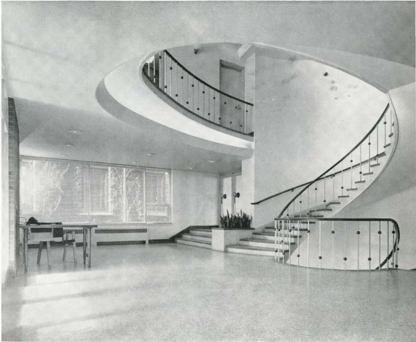
The main stair is illuminated by concealed fluorescent coves supplemented by pinpoint spots. West windows will eventually open to auditorium foyer. Doors to cafeteria show to left of stair.
