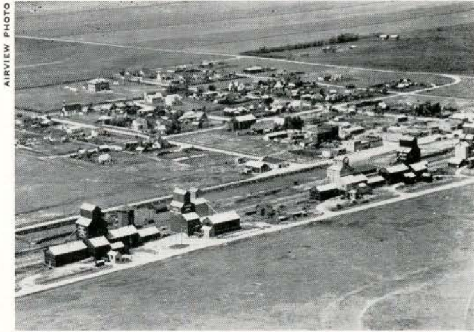
Granum, Alberta — Showing typical form of subdivision as well as the type of building in a small Alberta prairie town.
