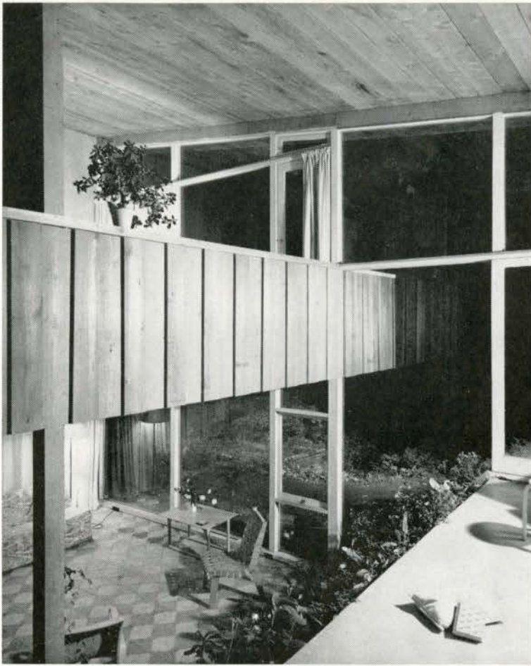
INTERIOR VIEW LOOKING SOUTH-EAST
