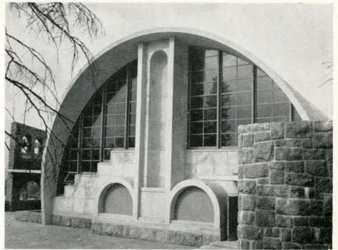
Fig. 2 Marial Chapel, façade. Facing of concrete and pink granite. To be completed by a 24' statue of the Virgin and bas-reliefs in the roundels.
