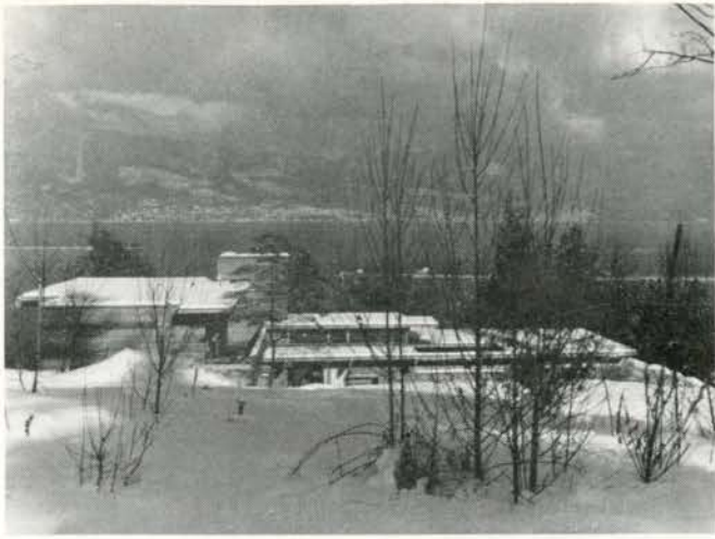
View from road towards North. Bedroom wing on left, living room clerestories to right of chimney mass, dining terrace and carport on right.
