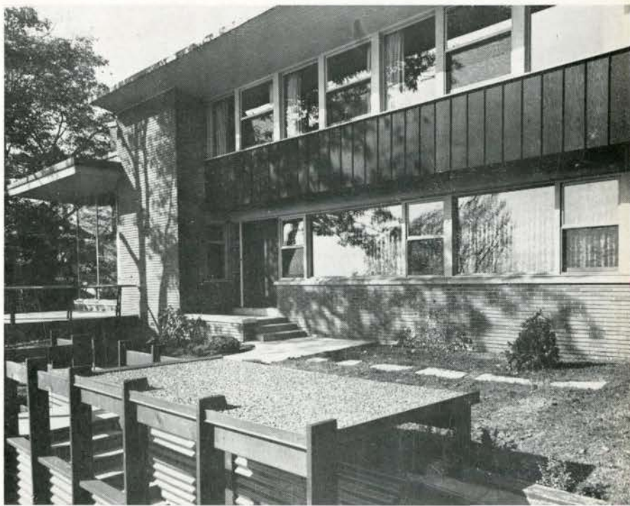
VIEW OF FRONT FROM ROOF OF CARPORT
