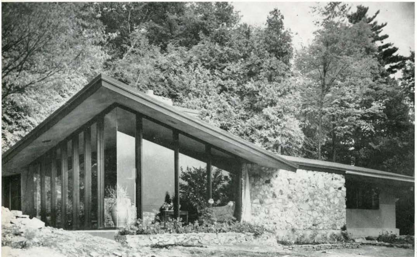
SOUTH-WEST CORNER OF LIVING ROOM
