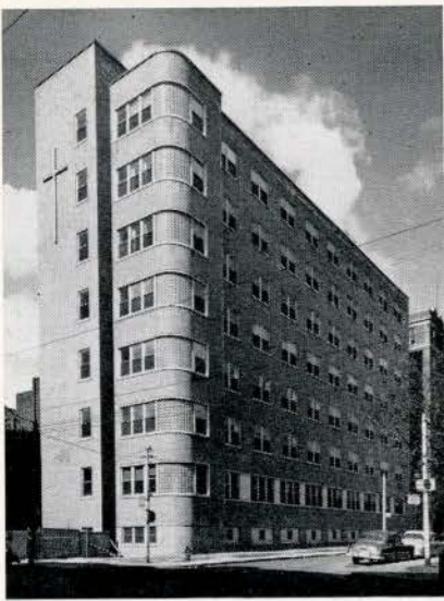
VIEW FROM S.E.
