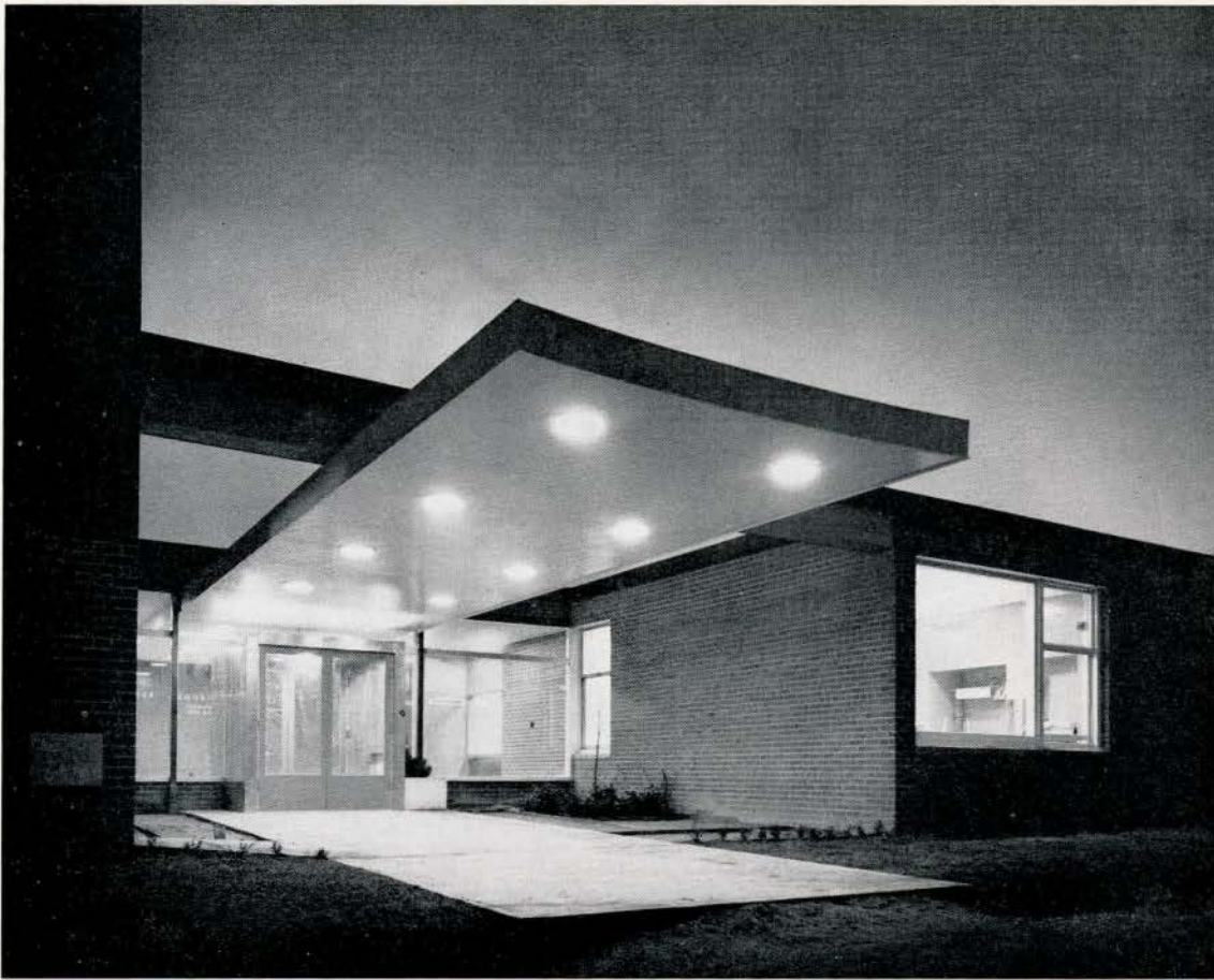
MAIN ENTRANCE CANOPY
