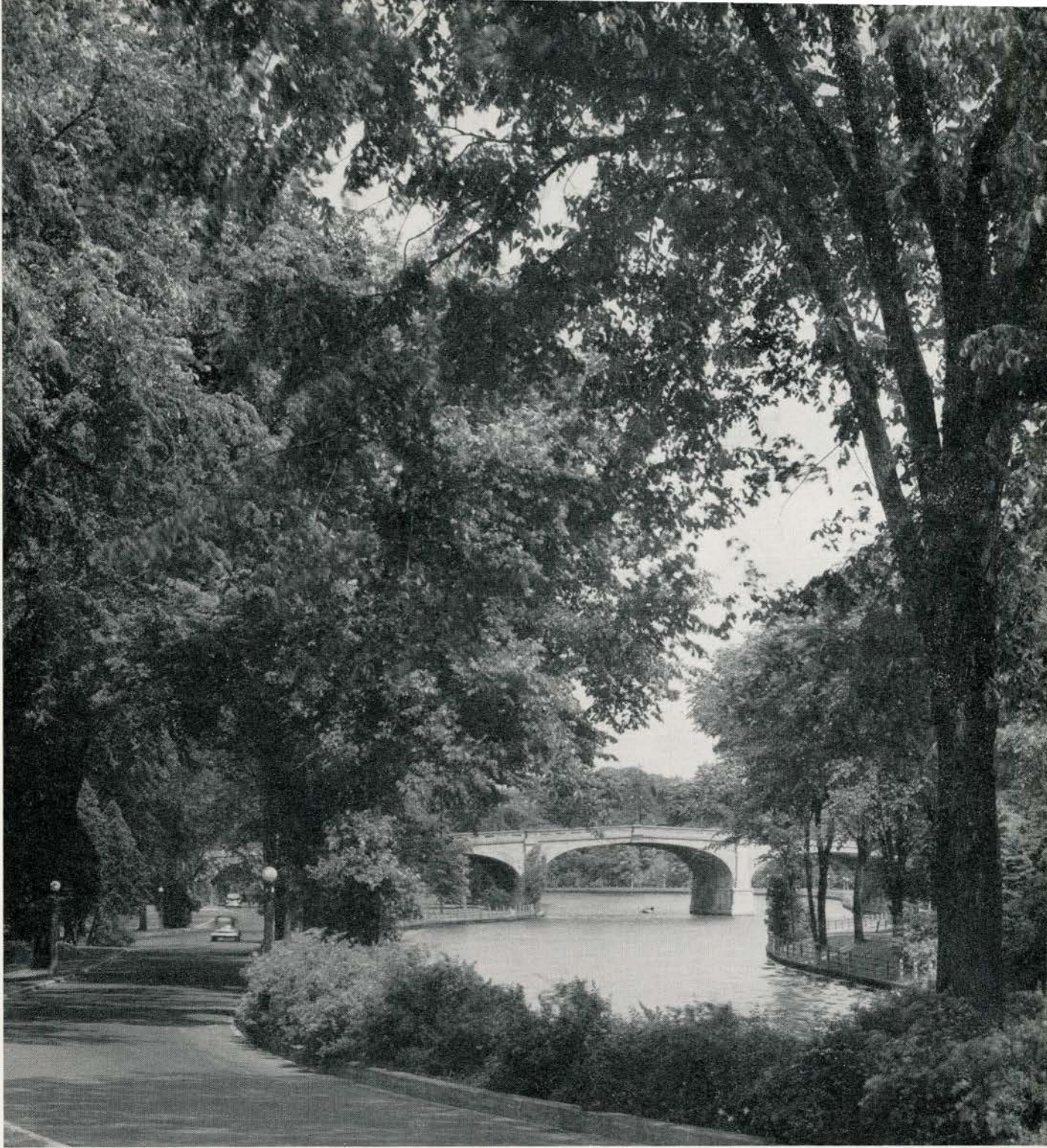
RIDEAU CANAL DRIVEWAY
