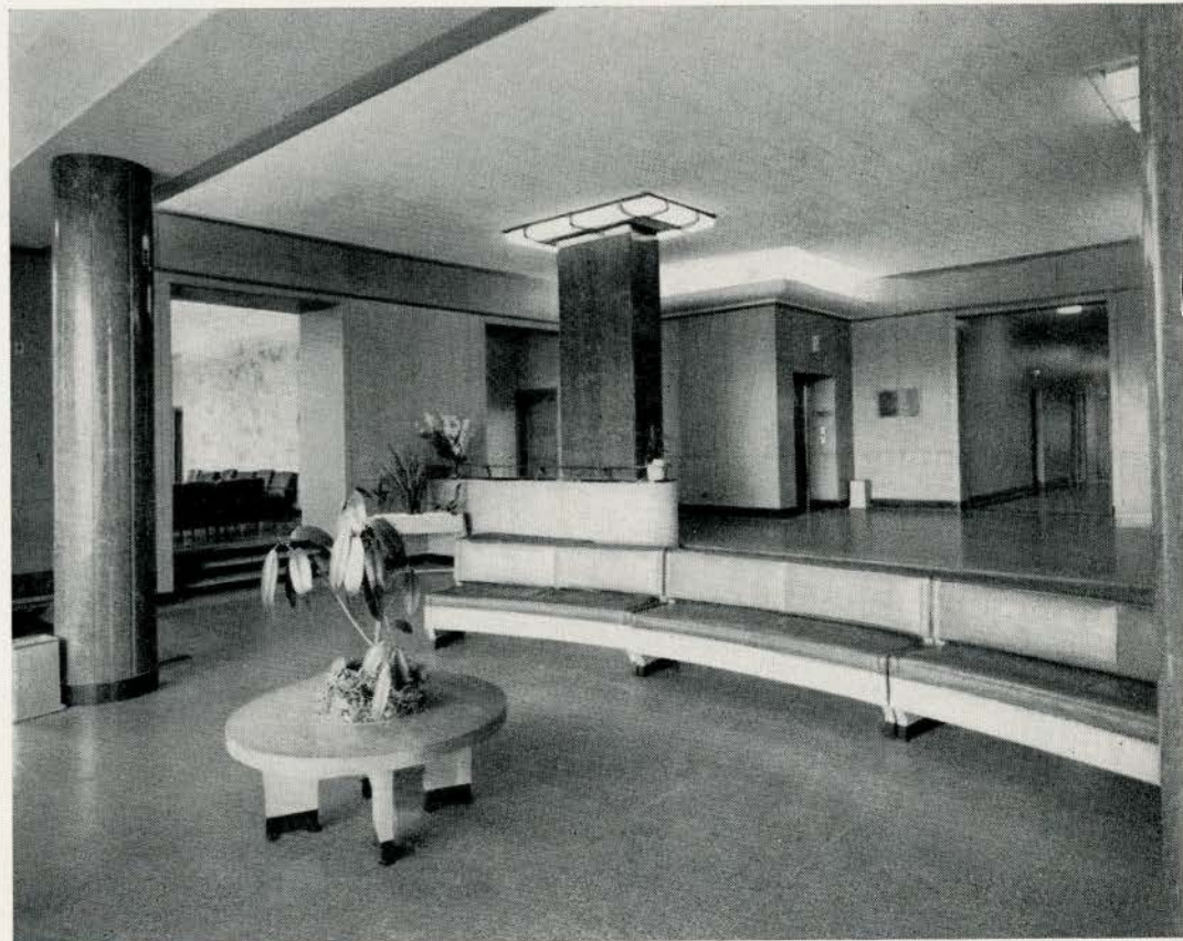
MAIN ENTRANCE LOBBY, ACTIVE TREATMENT BUILDING
