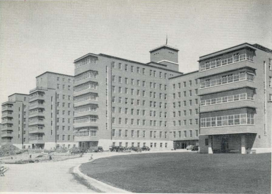
BUILDINGS FROM SOUTH-EAST
