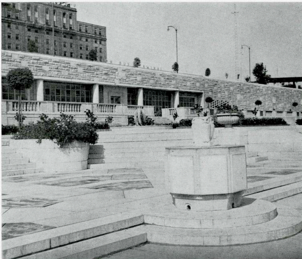
APPROACH TO BUS TERMINAL WAITING ROOM FROM RIVER ROAD DRINKING FOUNTAIN IN FOREGROUND BY ELIZABETH WYNN WOOD, A.R.C.A. W. L. SOMERVILLE, ARCHITECT DUNINGTON-GRUBB & STENSSON, LANDSCAPE ARCHITECTS
