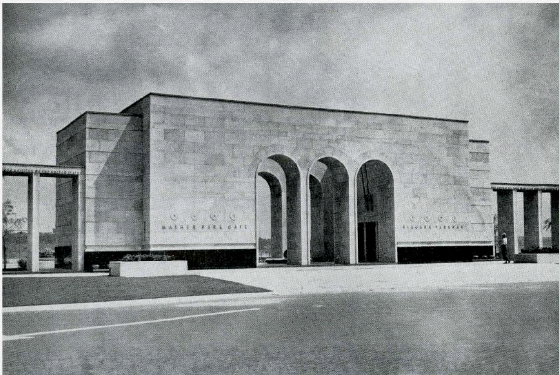
MATHER PARK GATE, MATHER PARK, FORT ERIE HUMPHREY CARVER AND CARL BORGSTROM, LANDSCAPE ARCHITECTS
