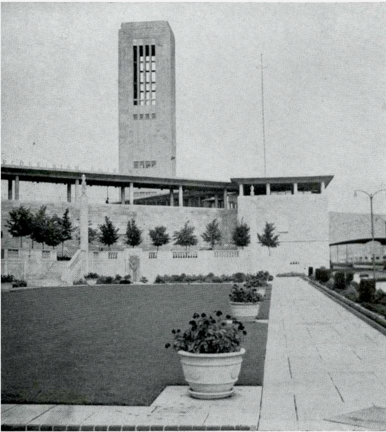
CARILLON TOWER FROM GARDEN BELLS WILL BE VISIBLE WHEN INSTALLED W. L. SOMERVILLE, ARCHITECT DUNINGTON-GRUBB & STENSSON, LANDSCAPE ARCHITECTS
