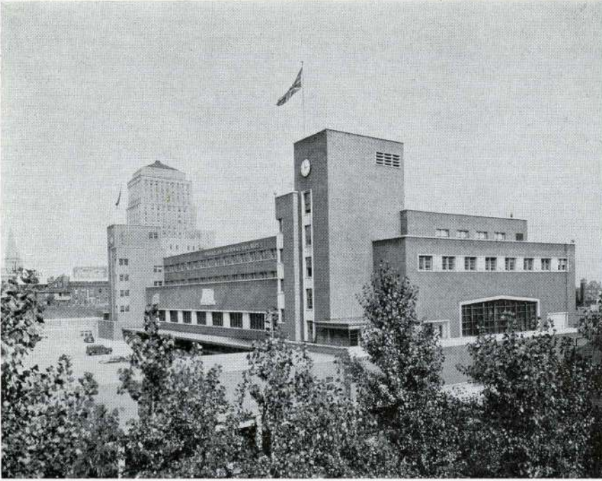
VIEW FROM MANSFIELD STREET
