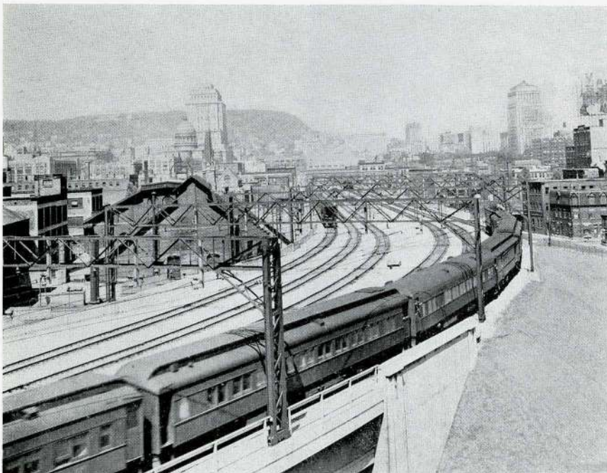
VIEW OF VIADUCT FROM WELLINGTON STREET LOOKING NORTH
