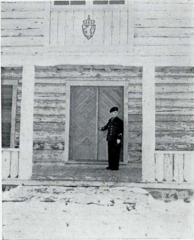
DETAIL OF MAIN ENTRANCE
