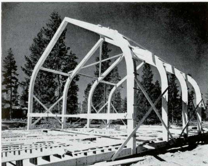
AN ARMY CHAPEL SHOWING FOUR ARCHES ERECTED OF 26 FT. SPAN
