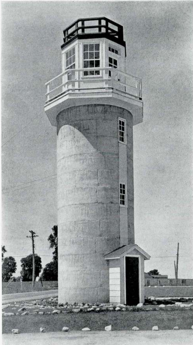
Air Force on one station has made use of an old farm Silo for special wireless equipment
