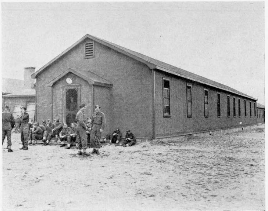
"A standard type dining hall and kitchen of lumber and tarpaper construction as built and used by the Canadian Army. The dining hut can accommodate 500 men at one sitting, 250 in each half of the building. The hut is considered of temporary construction."
