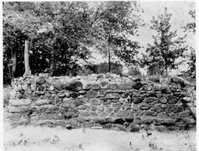
An exterior wall of the south west bastion, still standing to a height of four feet. Large and frequently uncut granite and limestone boulders are laid in lime mortar, without binder, and probably plastered on the inside surface. There is a rubble core, since the inside and outside stones do not overlap.
